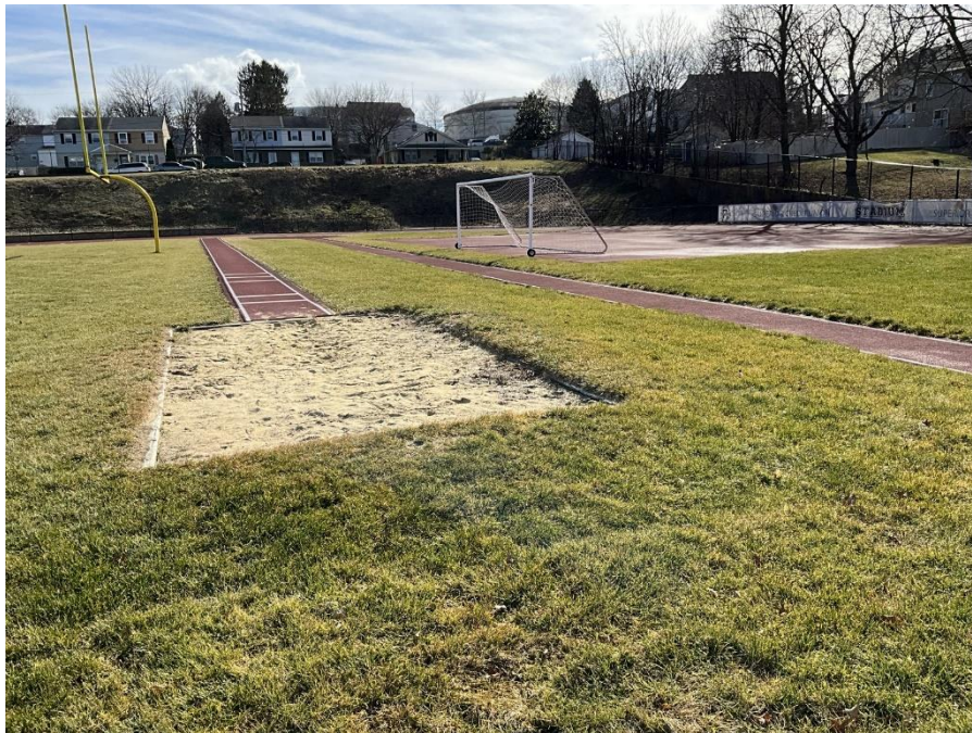
Photo 22 – Running Track – Jumping Venues Runways sitting low and staining visible in some areas (see pole vault runway at right); pit cover is missing. Surface in good condition.
