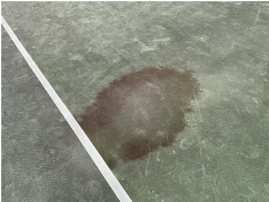
Photo 27 – Tennis Courts “Bird Bath” (low spot) on court with staining due to organics / pyrite. There were not many of these on the courts.
