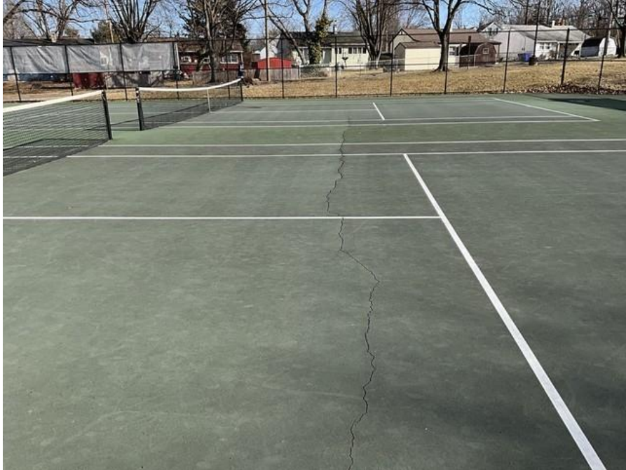
Photo 26 – Tennis Courts (Looking NE) Continuation of large crack. Heaving is evident.
