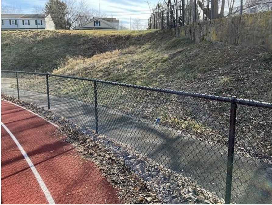
Photo 2 – Steep embankment at SW corner of stadium (Looking SE) Limited buildable area and maintenance issue / Fence within recommended 1-meter setback.
