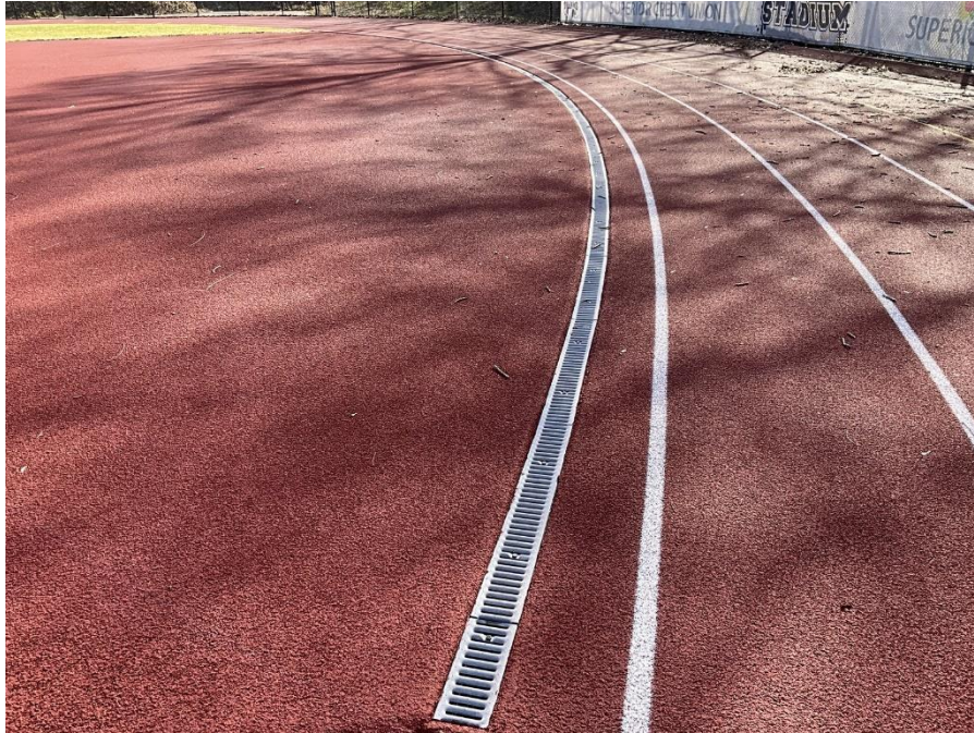
Photo 21 – Running Track SW radius; track surface in good condition; note organics (branches and leaves) along fence should be removed for can lead to staining.
